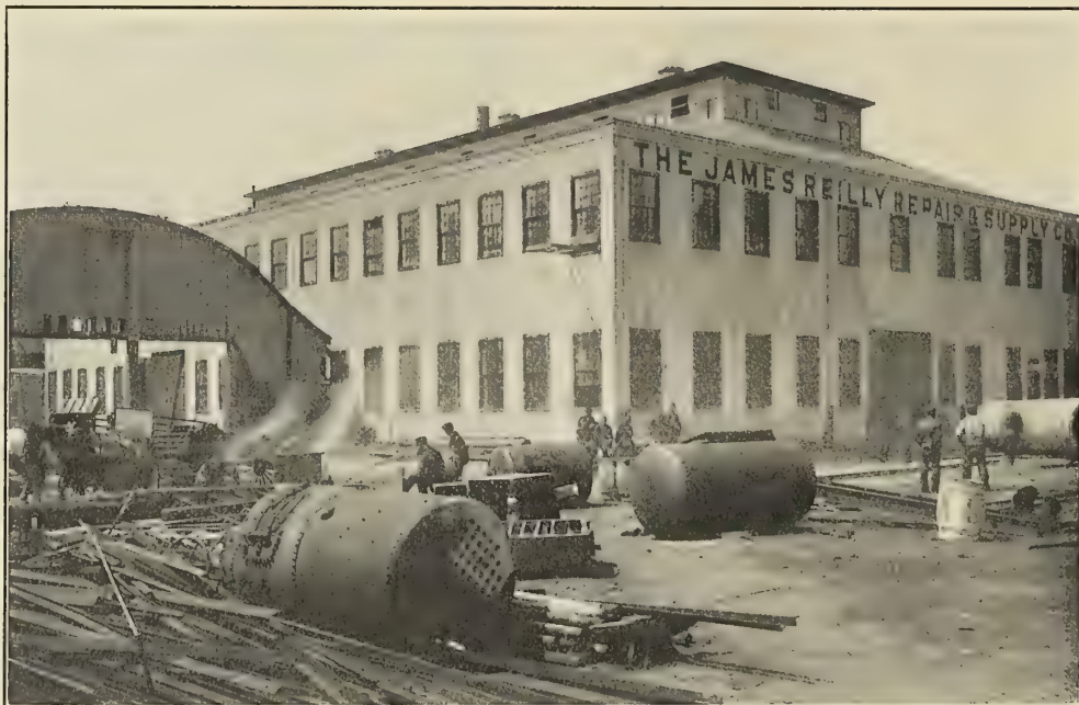
EXTERIOR VIEW OF THE JERSEY CITY REPAIR SHOPS.
